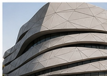
CURVED & COMPLEX SURFACES Seamless transitions and intricate curvatures made possible with GFRC.
